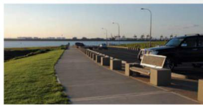
of materials. Concrete was selected because of its durability and minimal maintenance requirements. Nearly 600 pre-cast concrete elements were used in the project to form a suite of urban elements that include bollards, wheel stops, separation blocks and sections of kerb.
